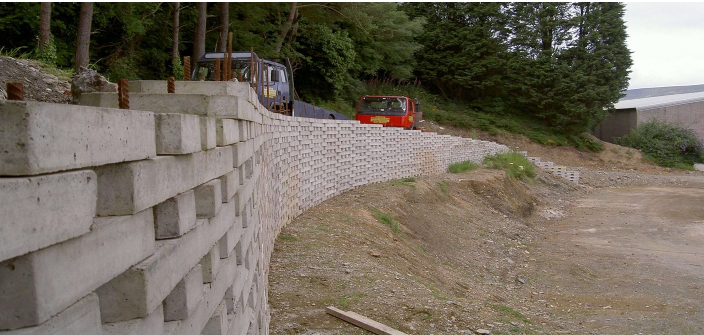
Access Road Walls
