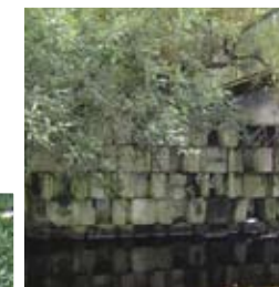
1000mm V Blocks constructed speedily to stop land slide and support a bridge in an environmentally sensitive location at the River Diggel in Oldham, Lancashire.
