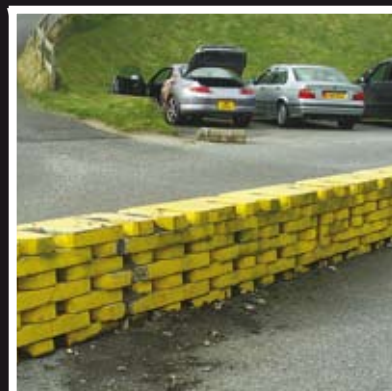
Wall straightened after collision.
