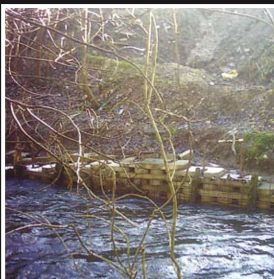
Low carbon W Blocks used as a rapid flood defence method in river bank enforcement.
