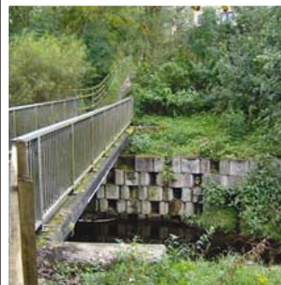
1000mm V Blocks constructed speedily to stop land slide and support a bridge in an environmentally sensitive location at the River Diggel in Oldham, Lancashire.
