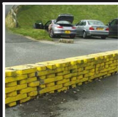
These pictures show an interlocking demountable W Cast wall after an impact.
