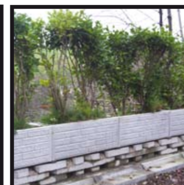
Instant W block wall Left, showing solar lighting for patio Right, with interlocking troughs.
