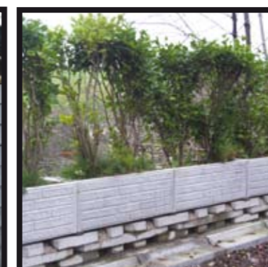
Instant W block wall Left, showing solar lighting for patio Right, with interlocking troughs.
